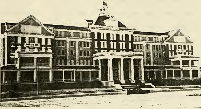
Plate 25: Main Block, East Elevation, 1985
